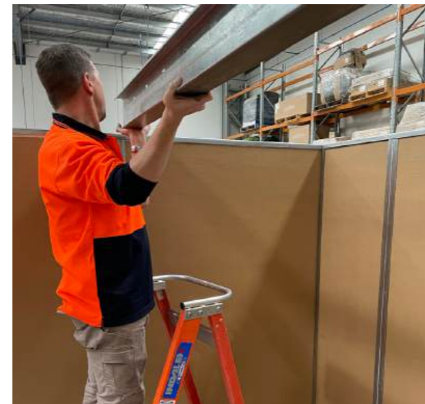
Series 2 Studio in construction
