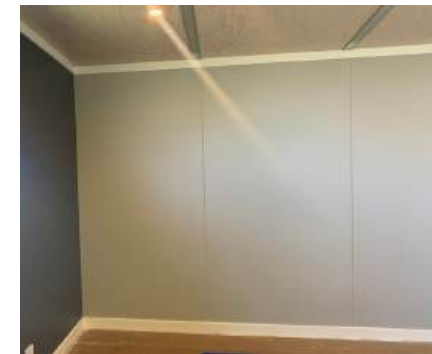
Durra Panel Painted Finish with panel to panel joints caulked with a flexible and paintable sealer
