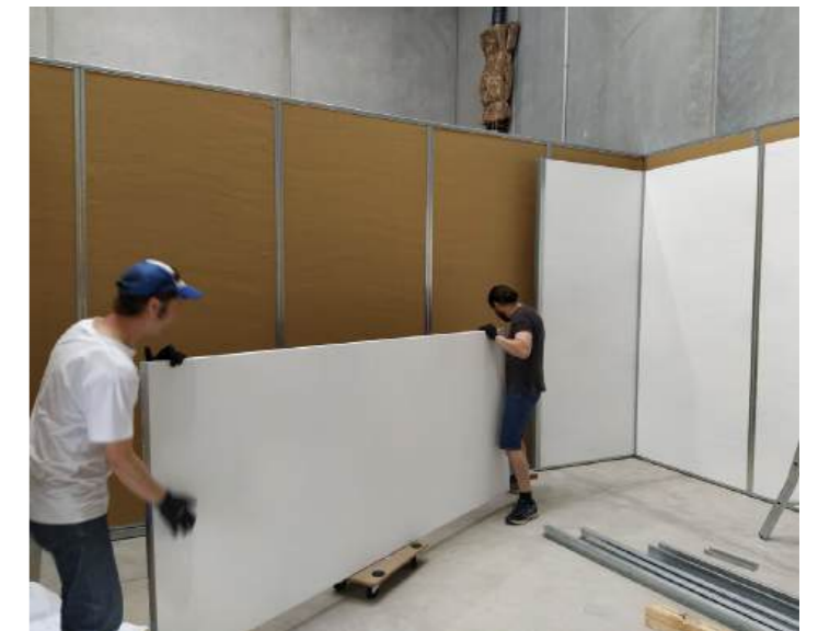
Series 3 Studio in construction
